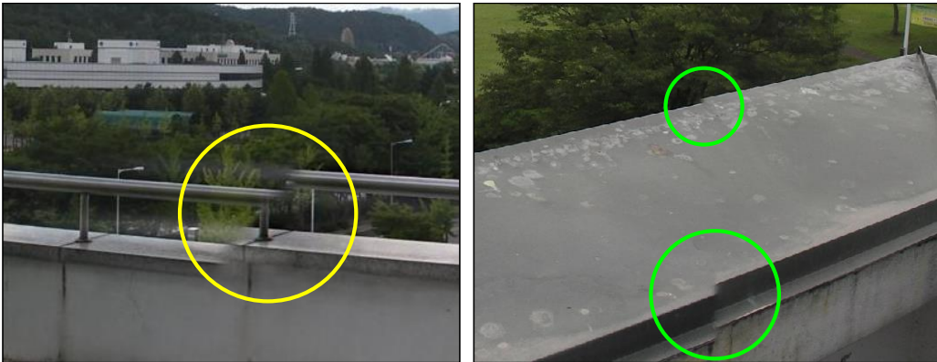
Fig. 1. Example of structure misalignments caused from parallax effects
